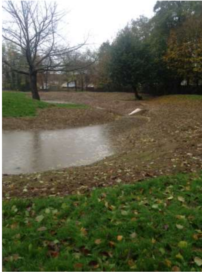
Plate 6 Flood storage attenuation basin in Fonthill Park, Southmead
