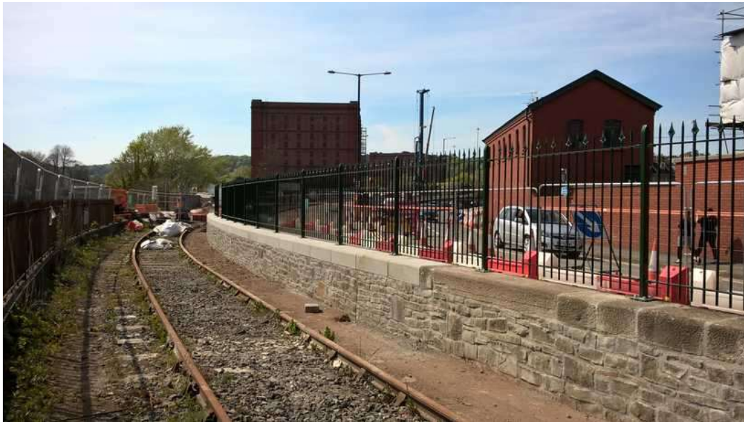
Plate 4 Cumberland Road flood defence wall
