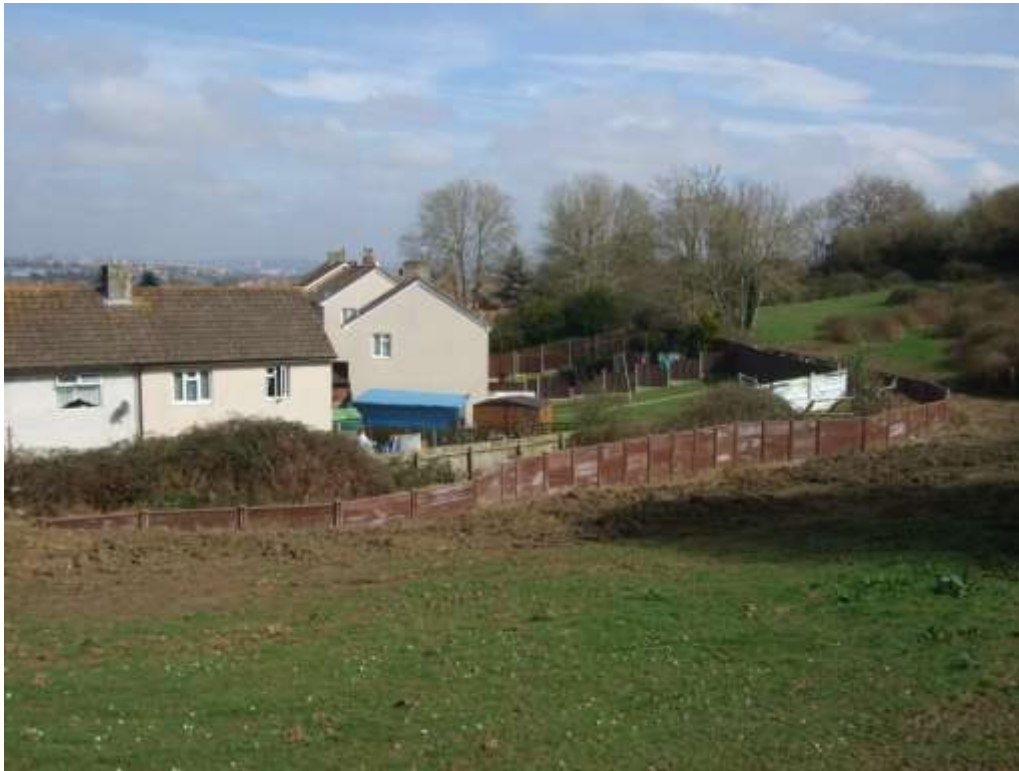
Plate 5 Flood proof fencing in south Bristol
